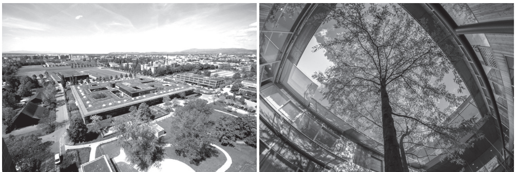
Fig. 1&2. REHAB Basel showing multiple courts and spherical skylights for special moods.
